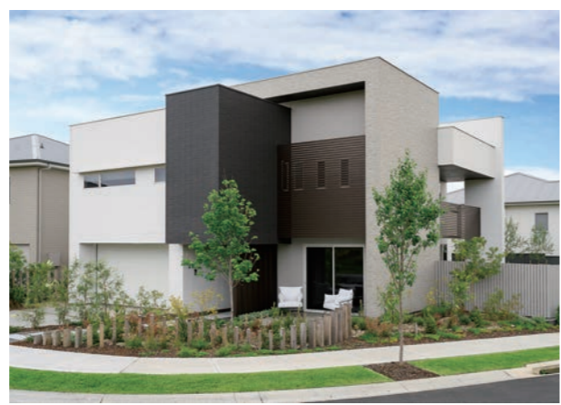
SHINKA House, a SHAWOOD project built to ZEH standards
