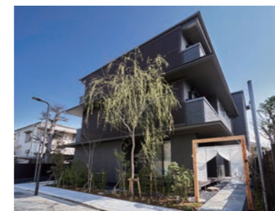
YANAKA SOW in Tokyo Hotel 3 stories totaling 680.55 m 2 . 13 rooms in total ZEB Ready (BEI: 0.45)
