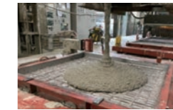
Feeding fresh concrete
