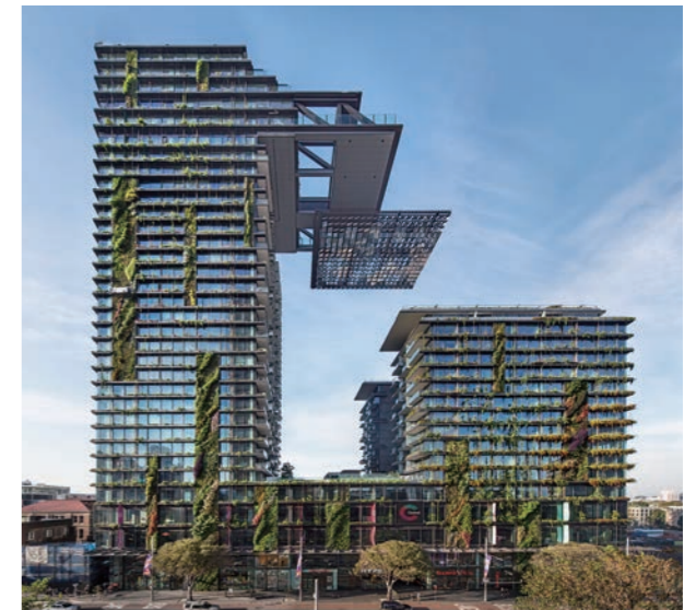
The Central Park Project features aerial gardens, impressive green walls, and reflectors to take advantage of natural light. In 2019, one of the project’s high-rise condominium buildings received the world’s highest award from the Council on Tall Buildings and Urban Habitat (CTBUH), having been evaluated as “world’s best” in both name and reality.
