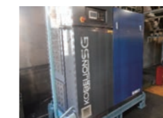
Upgrading compressors (steel plant)
