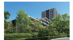
Grande Maison Water Purification Garden City Forest Gate, Chuo-ku, Fukuoka City
